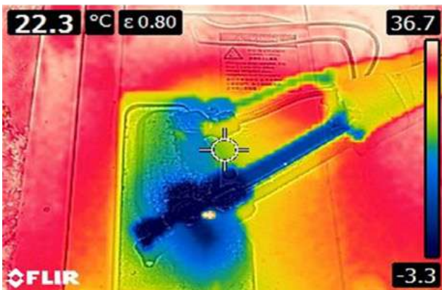
AC outdoor unit (standard and infrared camera) showing that extremities of the hose are not properly insulated
